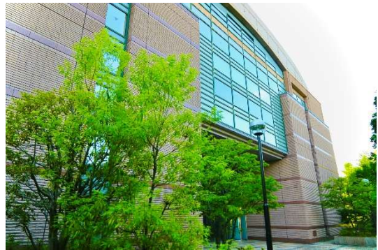
Exterior view of the new R&D Center building
