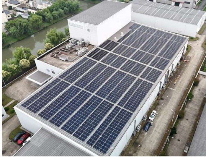
NIPPN (Shanghai Jinshan) Co., Ltd. with photovoltaic power generation facilities.
