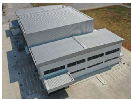
Exterior View of the Plant
