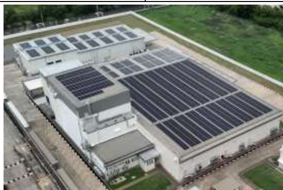
NIPPN (Thailand) Co., Ltd. with photovoltaic power generation facilities.
