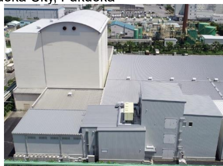
The newly constructed premix plant (lower part of the photo)
