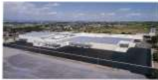
Second Isesaki Plant
