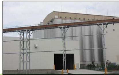
Loading facility for bulk carriers for shipping wheat bran at Chiba Mill
