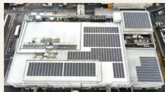
Ryugasaki Frozen Food Plant, with newly installed photovoltaic panels
